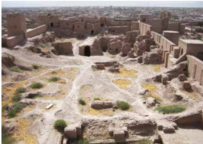
Fig. 98 Eastern upper citadel, restored walls and remains of Unesco-trenches, towards the courtyard with the vaulted pathway and western enclosure, 2008
