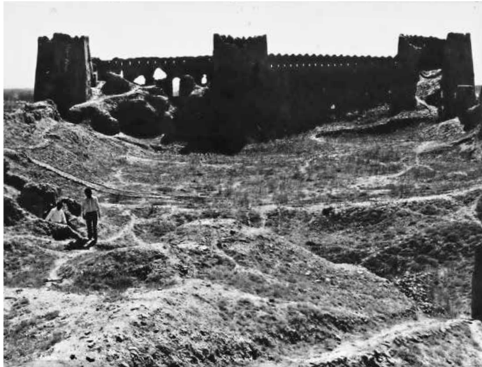
Fig. 96 Eastern courtyard, before restoration; from west, 1977 (courtesy Bruno/AKTC)
