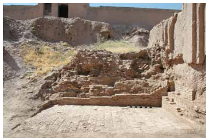
Fig. 101 Courtyard pavement and partly restored enclosure walls, 2005; from north
