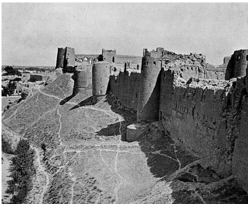
Fig. 309 Northern slope of the Citadel mound prior the Unesco restorations of 1976-1979 (Bruno 1976, 16)
