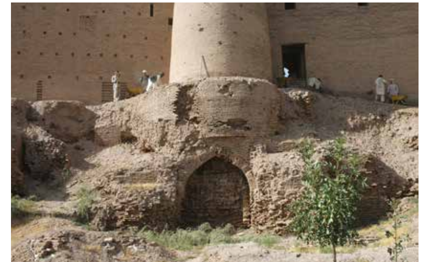
Fig. 310 Trench 3 before beginning of the excavation 2008, visible structures on the surface of the slope, i. e. a blocked pointed-arch gate and base drum of Tower XVIII; from north
