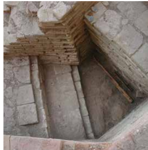
Fig. 391 Side entrance blocked by brick wall, edges of the steps originally stabilised by square timber
