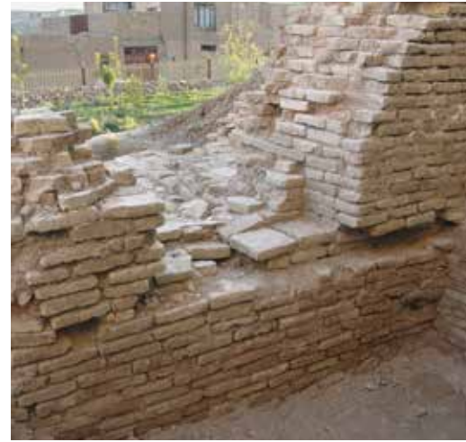
Fig. 395 Eastern tower, access from Room 3, recesses for square timbers to stabilise the stairs
