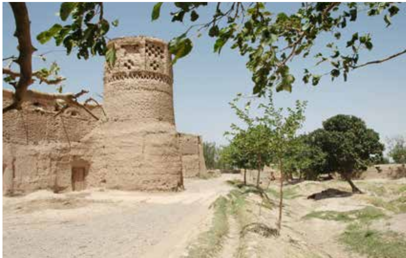
Fig. 513 Tower of contemporary fortified settlement ( qala ) in the Hari Rud valley
