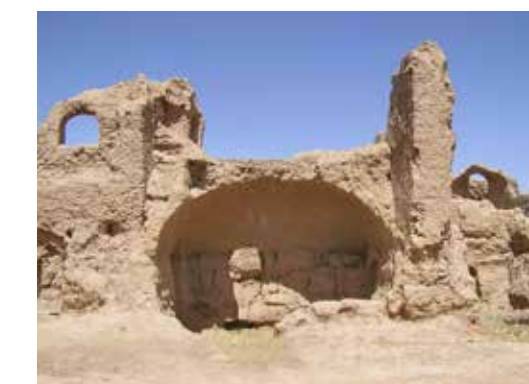
Fig. 1377 Ruins of two-storey mud-brick buildings
