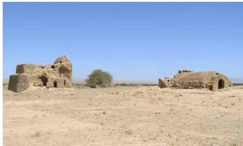
Fig. 1385 Historical ensemble with shrine Zn 4 (left) and cistern Zn 7 (right)
