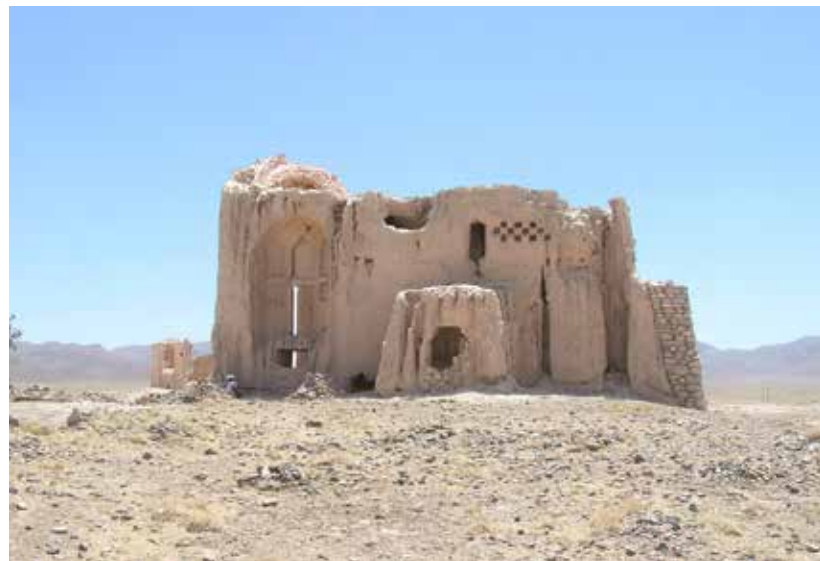
Fig. 1387 General view of the shrine, from north
