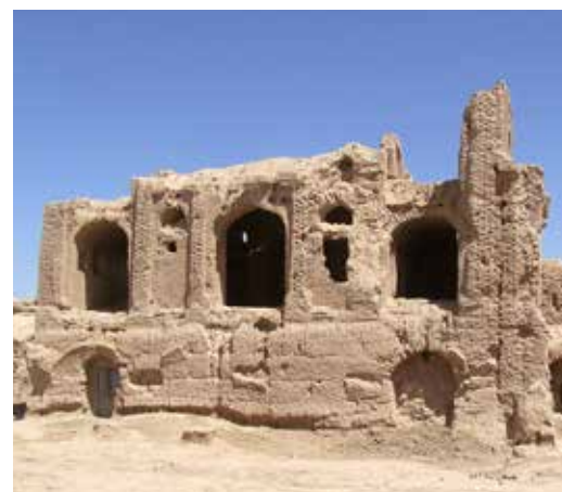
Fig. 1382 Ruin of a two-storey building
