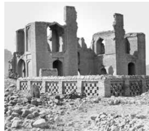
Fig. 1093 Northern façade in 1973 (Photo: B. O'Kane)
