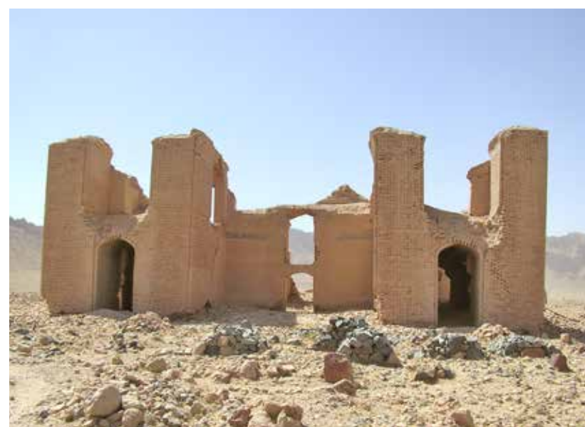
Fig. 1094 Northern façade in 2004
