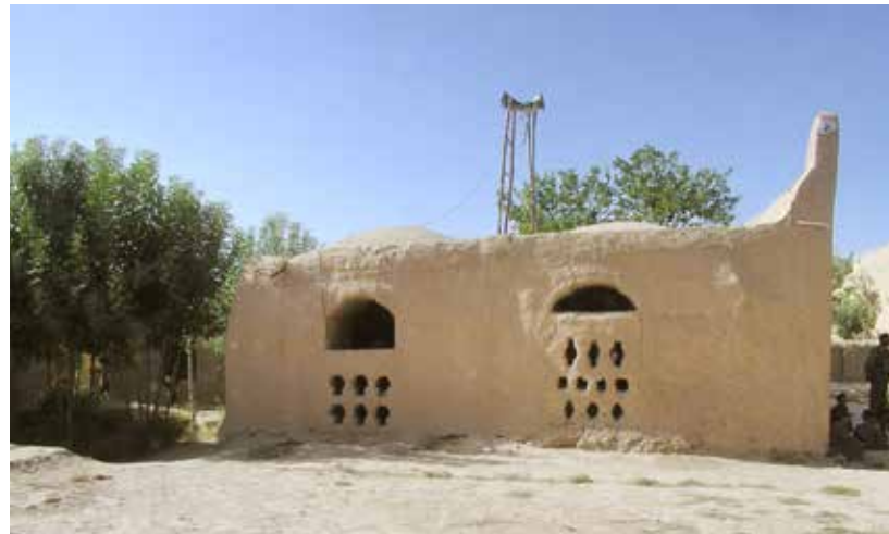
Fig. 484 Summer mosque, view from south
