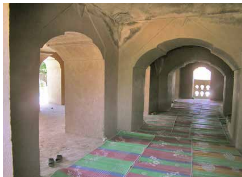
Fig. 487 Summer mosque, interior view
