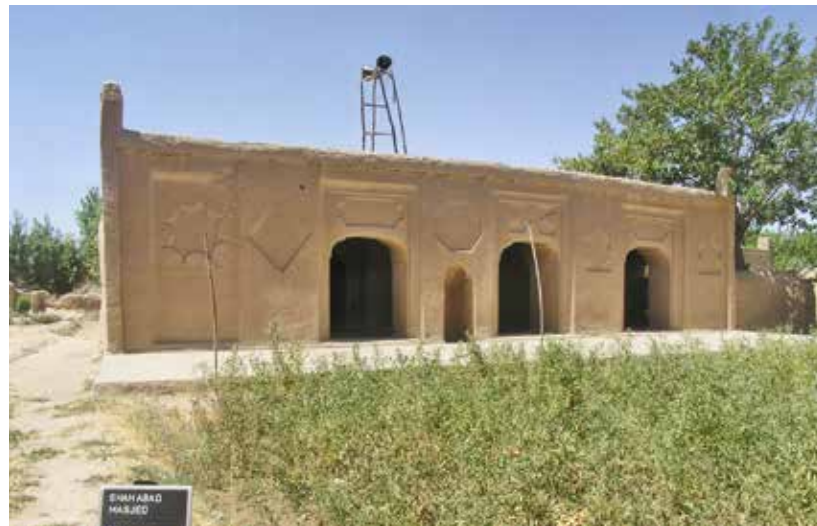
Fig. 485 Summer mosque, view from east
