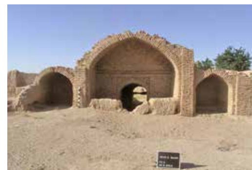
Fig. 478 The southern façade, from south
