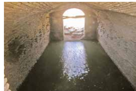
Fig. 480 Interior of the cistern, from south
