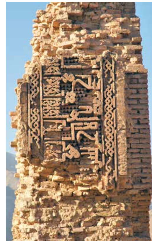
Fig. 101 Northeastern structure (CS 1b), detail of western brick decoration, from south
