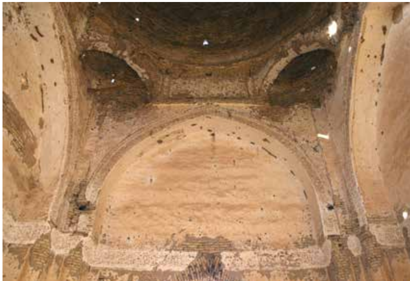
Fig. 95 Southwestern structure (CS 1a), inside view, from south
