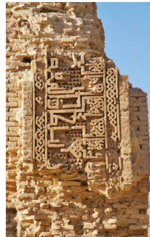
Fig. 103 Northeastern structure (CS 1b), detail of eastern brick decoration, from south
