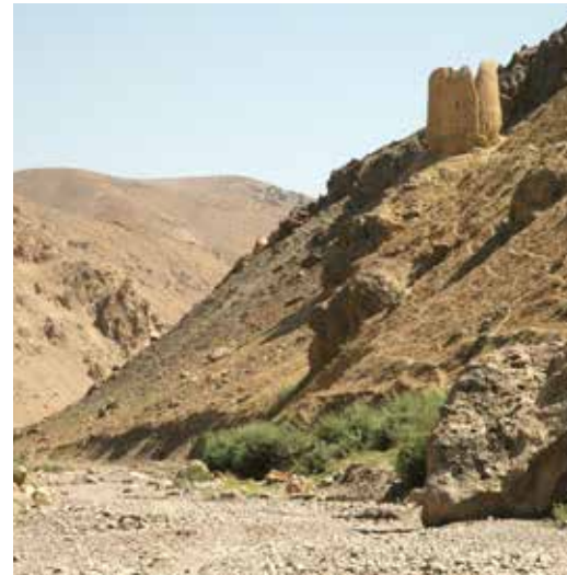
Fig. 71 Tower controlling a side vale (CS 28)
