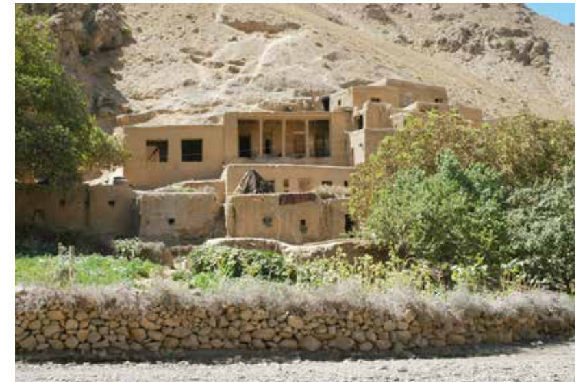
Fig. 69 Present-day houses with porches and large windows
