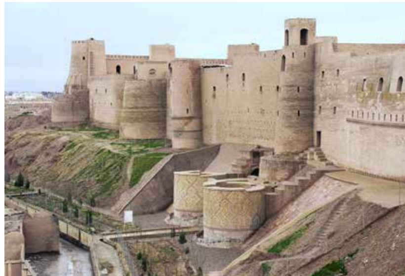
Fig. 565 Completed supporting structure, October 2009; from west
