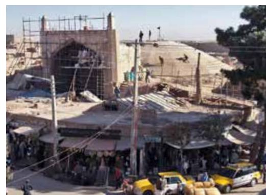
Fig. 783 Chahar Su cistern, during conservation (courtesy Archnet)
