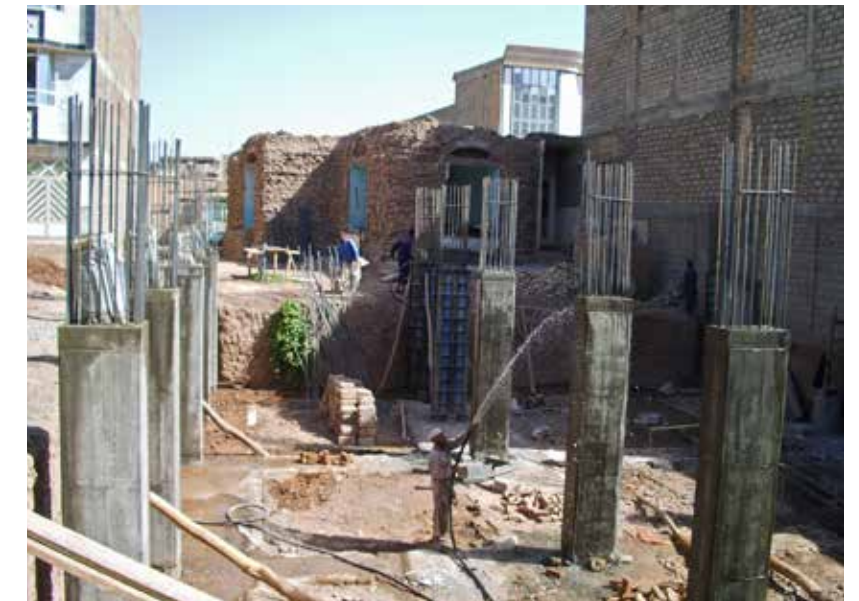
Fig. 769 Herat, construction zone, spot 27 (photo: B. Mutin).
