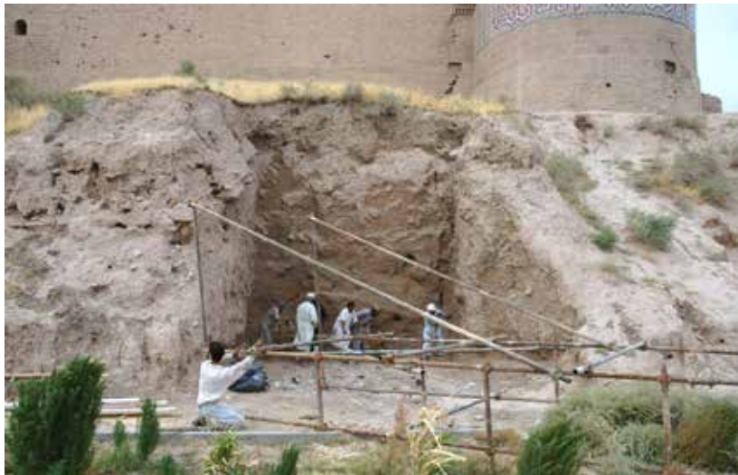
Fig. 277 Trench 2, cleaning of the surface and construction of scaffolding; from north
