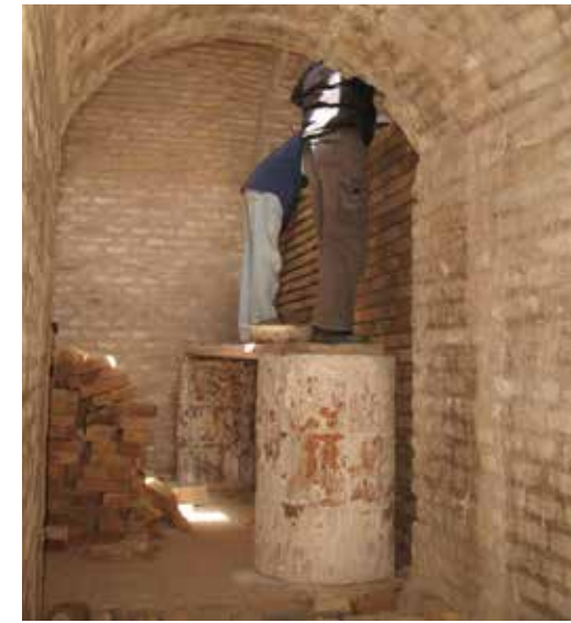
Fig. 8 Removal of a wall in the magazine
