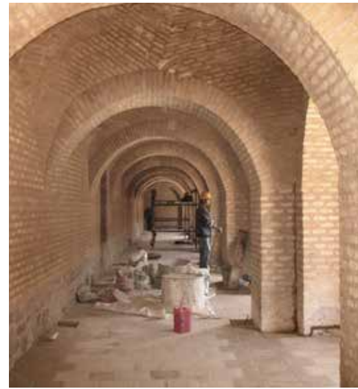
Fig. 5 Ground floor: work in progress
