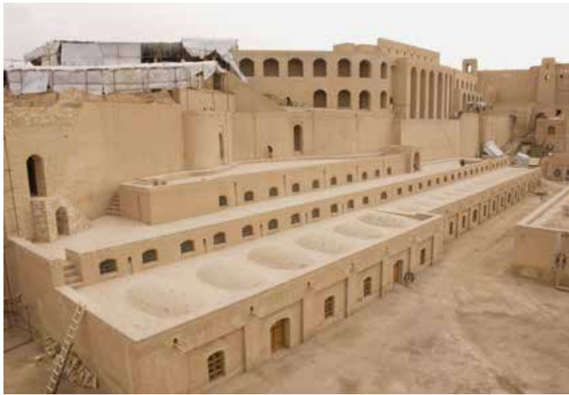
Fig. 4 Structural improvement in progress
