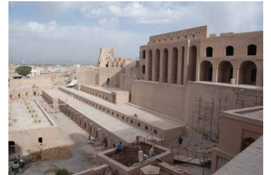
Fig. 8 Restoration work in progress, 2009
